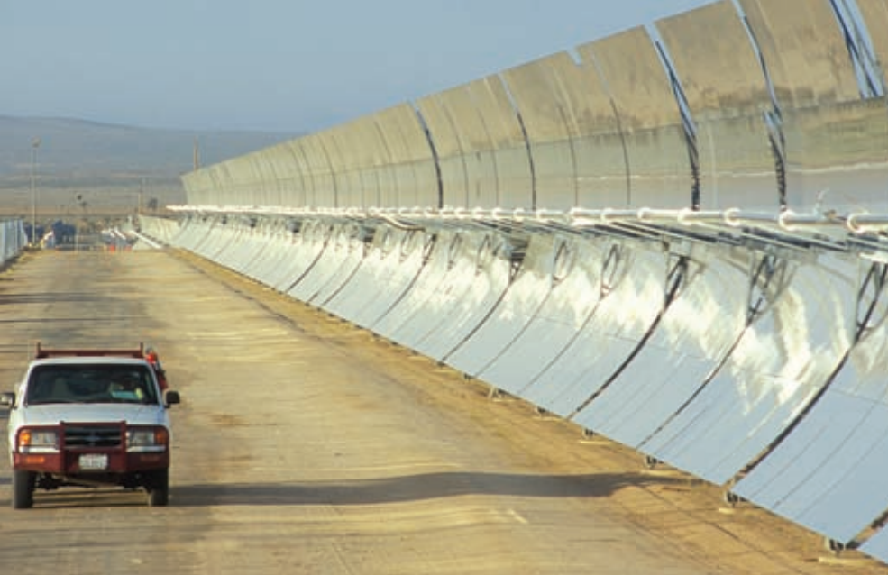
A solar field, part of Kramer Junction Company's Solar Electric Generating System, in Southern California's Mohave Desert. The parabolic mirrors heat an oil that makes steam to run turbines.
